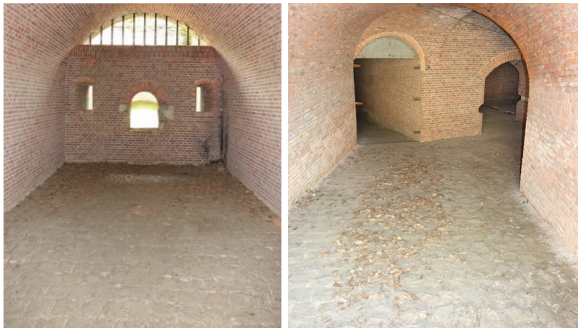
afb. 222: Vloeren in originele kasseien in gallerijen - periode periode 1859 - 1894 /. 2018. © ORIGIN
