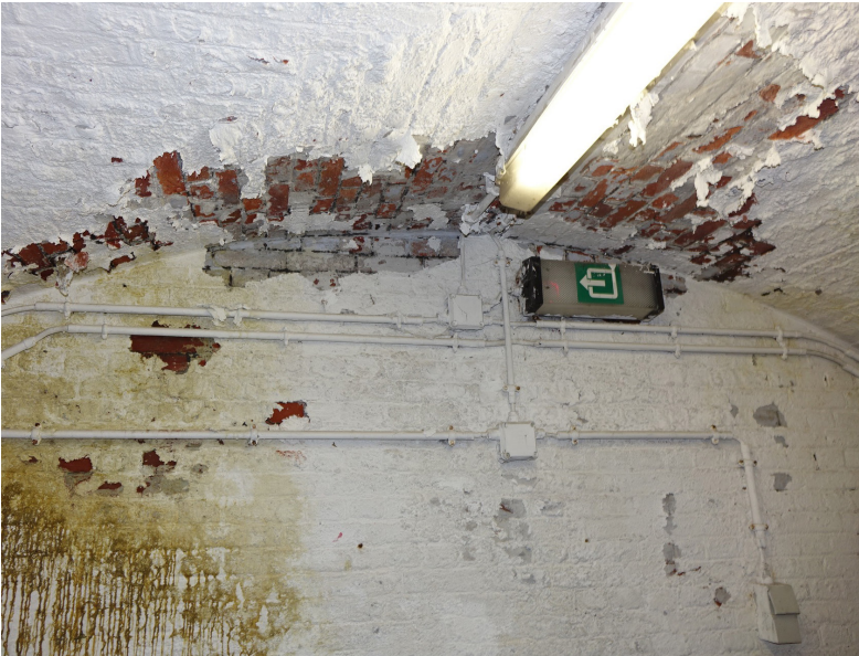
afb. 173: Afbladderende verf interieur courtine 3-4 © Origin
