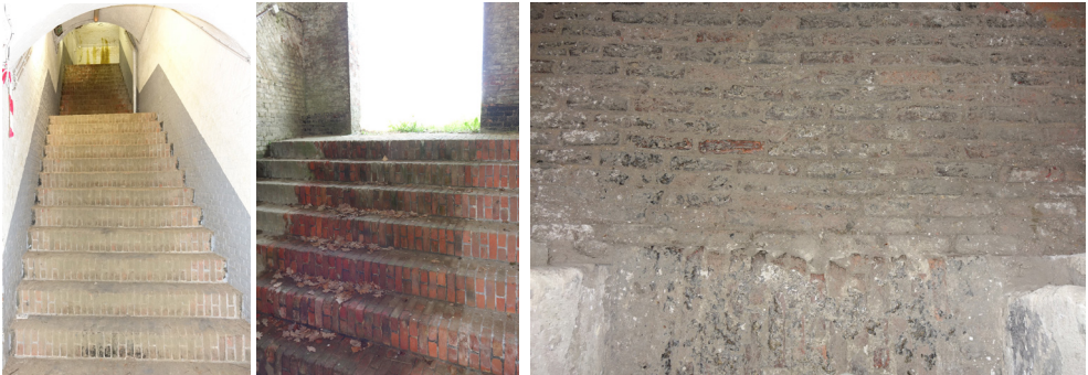
afb. 218: Trap naar dakkapel (travers) - bovenop de courtine) in origineel metselverband - periode 1859 - 1894 / 2018. © ORIGIN afb. 221: Vloer in originele baksteen- periode 1859 - 1894 /. 2018. © ORIGIN
