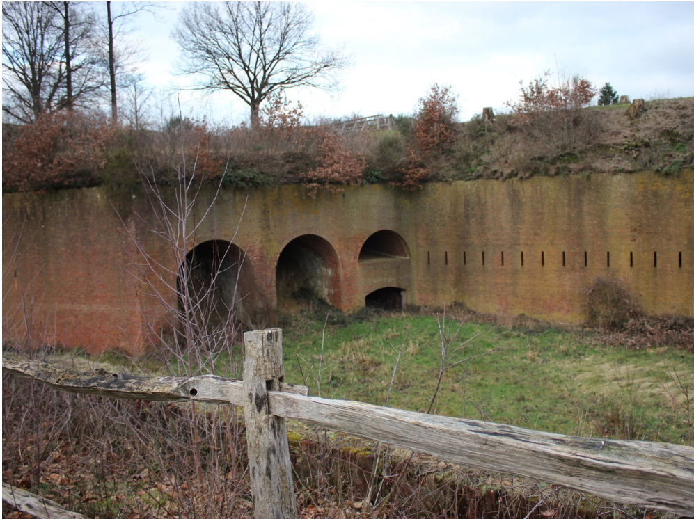
afb. 67: Chasseloup systeem van bastion 4 © Origin
